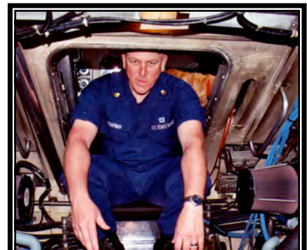
BM1 - Dave Chapman inside engine room of CG47218
